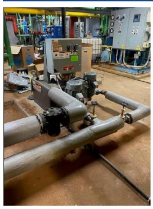
Last week, Utilities and Energy Management Distribution team completed work replacing a steam condensate receiver in the Health Science Research Building (HSRB). The new unit (left) replaced an existing unit which was beyond repair (right) and is expected to deliver annual savings of approximately \$28,000! Say what!? How does that work? UK uses two fossil fuels (natural gas and coal) to boil
