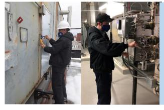
With a polar vortex bearing down on the region this week, our **Area Maintenance** teams doubled down on making sure buildings and equipment are ready for the cold. Far left, **Brian Gess** troubleshooting an air handler at Chemistry Physics. Left, **Bryan Poe** installing a new steam gauge at Jacobs Science Building. Right, **Lance Dunn** performing a maintenance check on air handler controls at Chemistry Physics.
