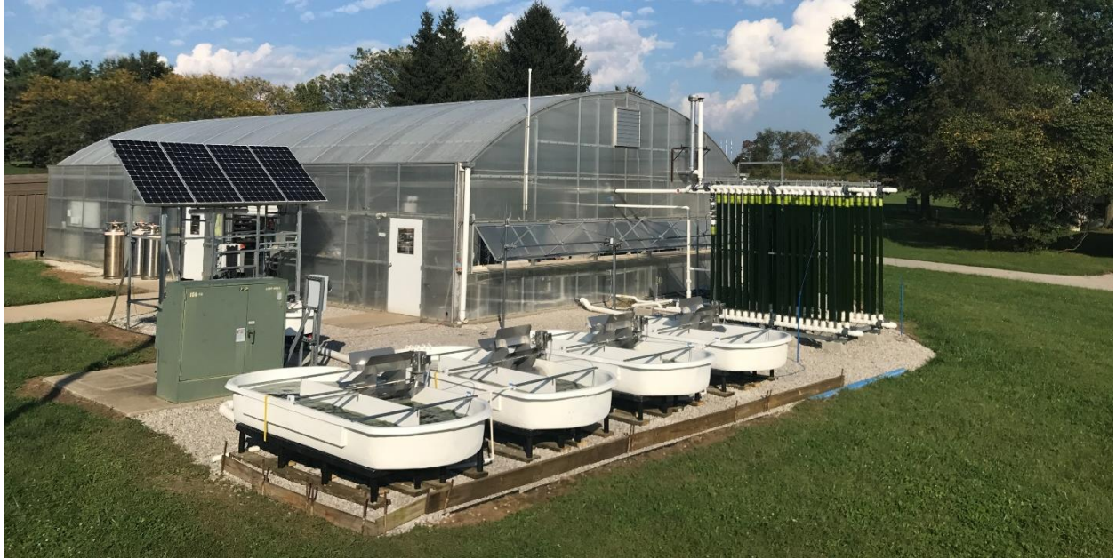
Figure 5: Expanded facilities at CAER Algae Greenhouse, Fall 2017
