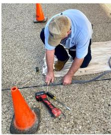
It may not feel like it now, but colder weather is on the way. Getting ready for winter, **Clyde Durham**, Area 1 Maintenance Tech, seals gaps between concrete panels in the plaza between Whitehall and Patterson Office Tower (left). Resulting from age and weather, these cracks allow water to penetrate the basement ceiling of the connector tunnel between the buildings.
