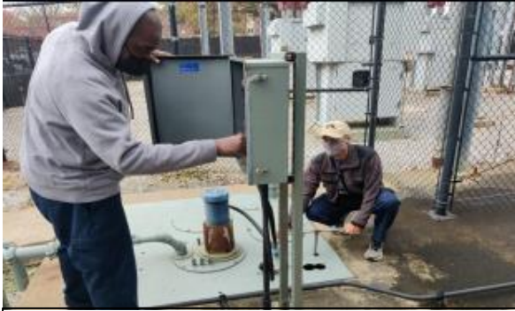
Corey Chenault and Henry Huffines draining a cooling tower pump sump
