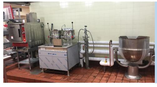
The steam kettles in the kitchen of Good Samaritan, Lexington's oldest hospital, were in need of renovation and upgrade. Under the direction of UK Facilities Management Medical Center project manager Josh Tarter and superintendent Eddie Spencer, the rusted piping, valves, and steam traps were replaced and the original kettles were relocated to make way for new kettles. The equipment was also repositioned to better exhaust steam from the kitchen. EXCELLENT WORK!
