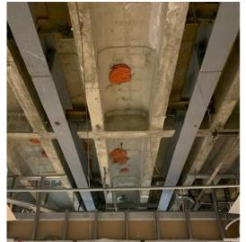
CT scanners are very heavy pieces of equipment (2-3 tons), so the floor underneath must be strong enough to bear this weight. Sometimes this requires installation of structural reinforcement in difficult to reach locations. A new CT scanner was recently installed directly above the Chandler Hospital gift shop (right). Facilities Management Medical Center's project manager Jamie Carpenter and superintendent Eddie
