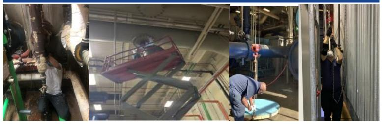
**Facilities Management's Utilities and Energy Management** teams were busy last week cleaning and performing preventative maintenance on our heating and cooling plants. At left, **Joe Flannery** cleans a flange at the Singletary Center. Second from left, **Henry Huffines** clears a condenser dirtleg. Second from right, **Cory Chenault** removes the head on Chiller #5. At right, **Steve Monroe** readies a steam valve for inspection. GREAT WORK UEM.
