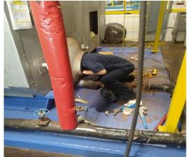
**Utilities and Energy Management** continues their efforts to ready campus heating systems for the cooler weather ahead. At left, **UEM's Paul Brooks** cleaning the mud drum on CUP boiler #1. At right, inside the
