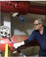
Utilities & Energy Management's (UEM) Heating and Cooling Plant teams were busy last week with steam system improvements. At left, Steve Monroe brings steam back up in the Central Utility Plant (CUP) after the installation of a new 20" line out of the plant. At right, Cory Chenault installing a new steam pressure reducing valve in the basement of Cooling Plant #2. UEM's three heating plants provide the steam needed to heat most of the campus.
