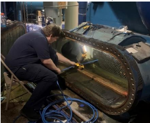
Joseph Harris jetting/brushing tubes on Chiller 2.
