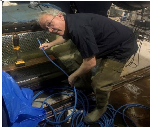
Steve Irvin jetting/brushing evaporator tubes on Chiller 2.
