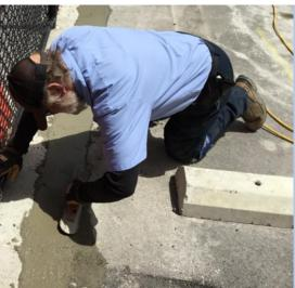
Last week, Curtis Crump (left) and Stuart Leasor (right), from CPPD Central Shops, cut a trench to install conduit for new automatic gates at the Central Utilities Plant. This is part of ongoing work that Utilities and Energy Management is leading to improve conditions for accessing our central plants to safeguard our capacity and deliver uninterrupted electricity, chilled water, steam, domestic water, and sewer services to campus facilities.
